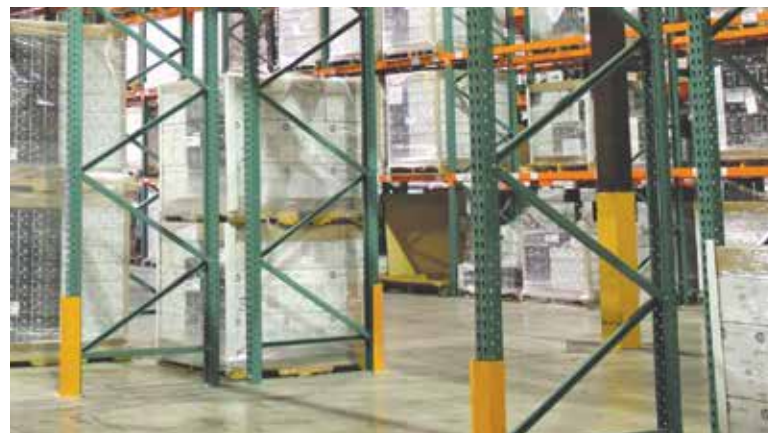
Bracing Arrangements in Uprights
